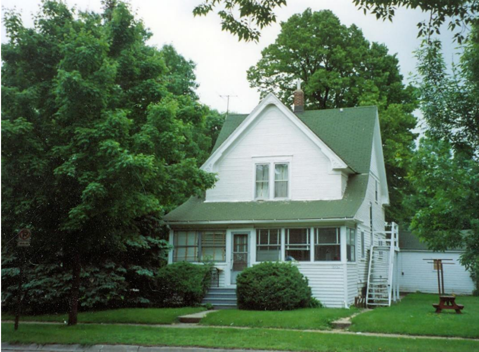
Duncan and Esther's home at 1343 Ellis Boulevard, Cedar Rapids. Like most houses in the Time Check neighborhood of Cedar Rapids, this house was severely damaged in the 2008 Cedar Rapids flood and was torn down soon after.
